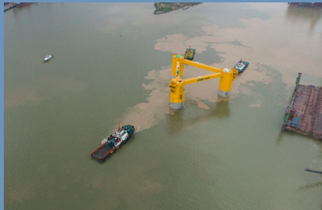
"FUYAO" departs Dongguan Yard prior to installation
