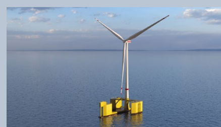
Trivane at 6m draft for assembly and tow
