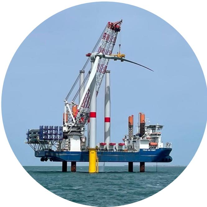
France is currently one blade short of having its first commercial offshore wind turbine as the team on board the vessel *Vole au vent* is completing the installation of the first GE Haliade 150-6MW unit at the Saint-Nazaire offshore wind farm site.
