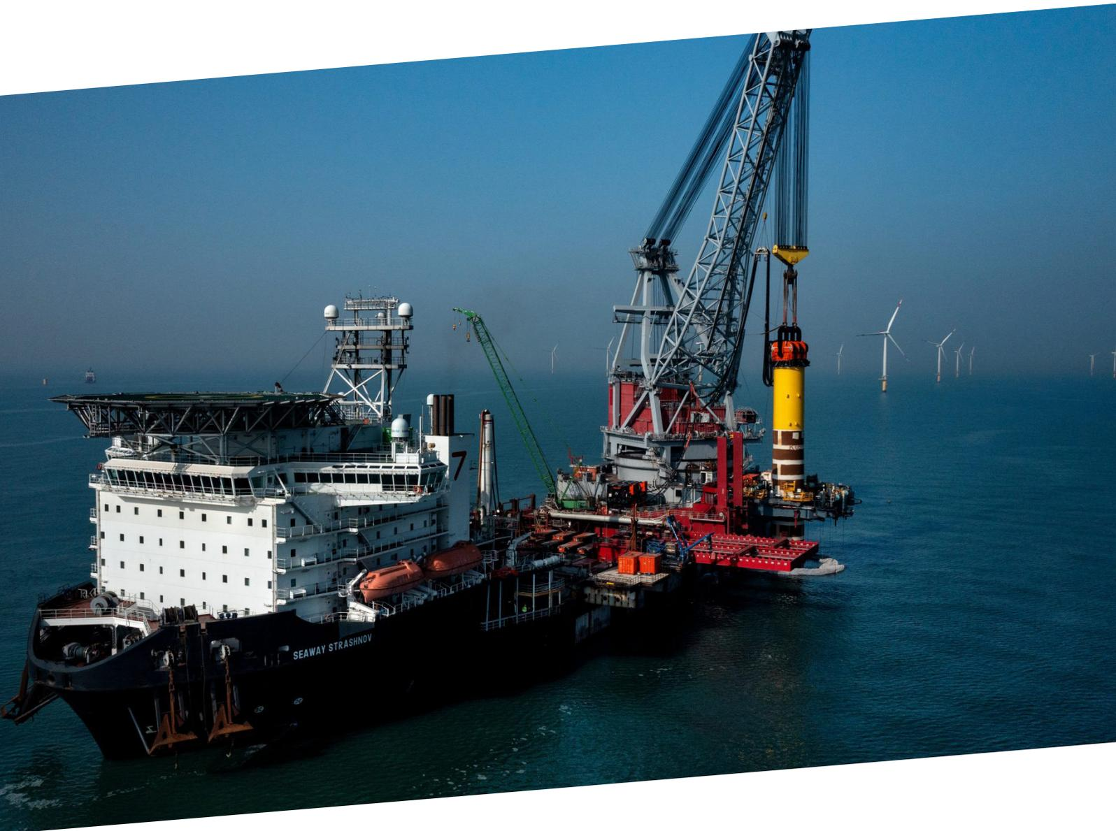
Seaway 7 also utilised innovative vibro pile driving technology to reduce underwater noise emissions, benefiting the marine environment in particular. We have achieved this together with CAPE Holland, who built and provided the world's largest Vibro Lifting Tool for the project.
