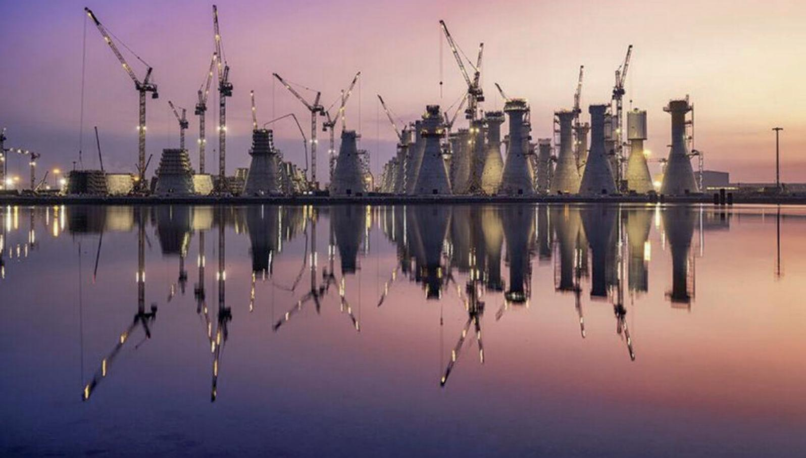
Bouygues Travaux Publics is in charge of the construction of the 71 gravity foundations on which the masts of the wind turbines of the Fécamp Offshore Wind Farm will rest.
