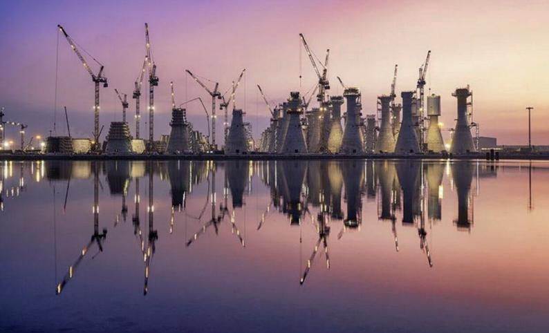
Bouygues Travaux Publics is in charge of the construction of the 71 gravity foundations on which the masts of the wind turbines of the Fécamp Offshore Wind Farm will rest.
